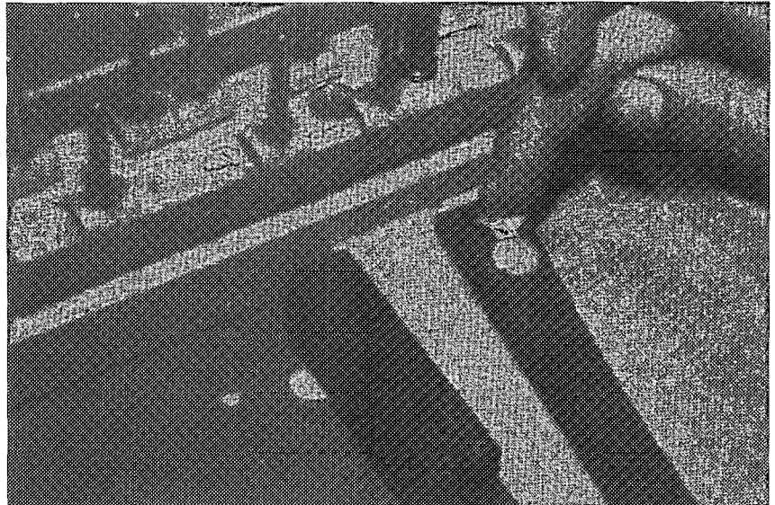
#10-11. This crack was not serious enough to have to drill the plug out and fix crack and replug. We repaired it by gluing it up and clamping it overnight. Those are two pieces of wood left and right to brace the repair. A folded piece of newspaper is placed between the surfaces on the right where glue may seep out and try to glue the brace wood to the support wood. The braces are later removed and the newspaper sanded away to clean up the repair. □
